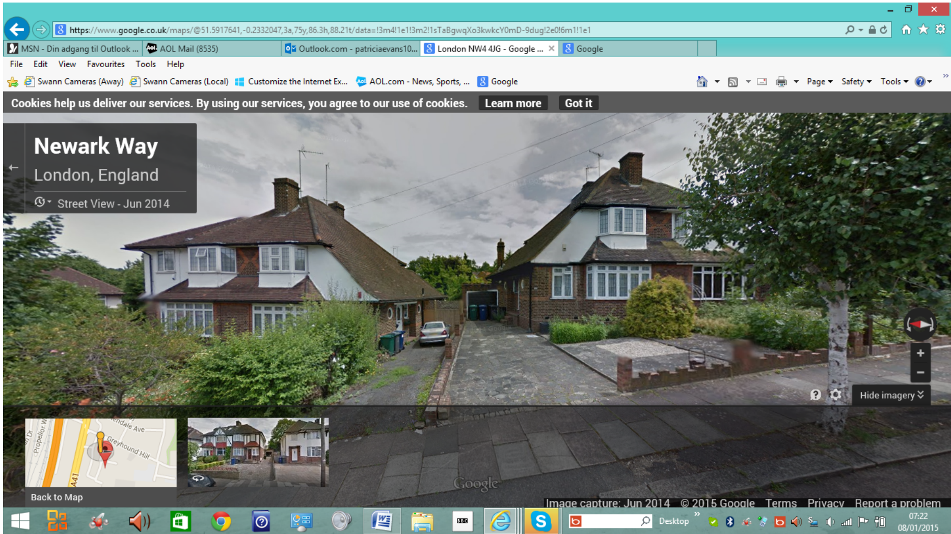
A pivotal photo: PRIOR to ALL works in 2014. H/03014/14 built the 2nd roof extension and 2nd roof extension with dormer. Photo date 8 January 2015 .
